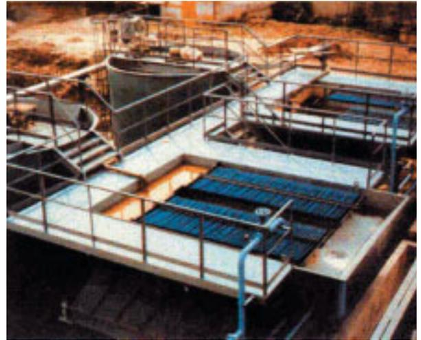
Installation in India of 2 x 100% lamella clarifiers with flocculation tanks. Each clarifier is rated for a maximum flow of 240 m<sup>3</sup>/h
