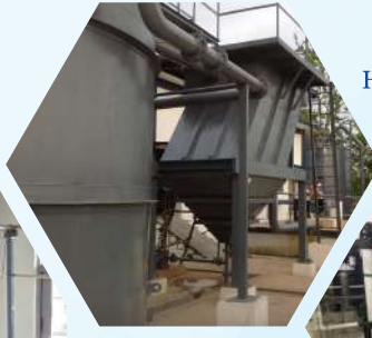
Lamella Clarifier at Air Force Station, Digaru, Assam
